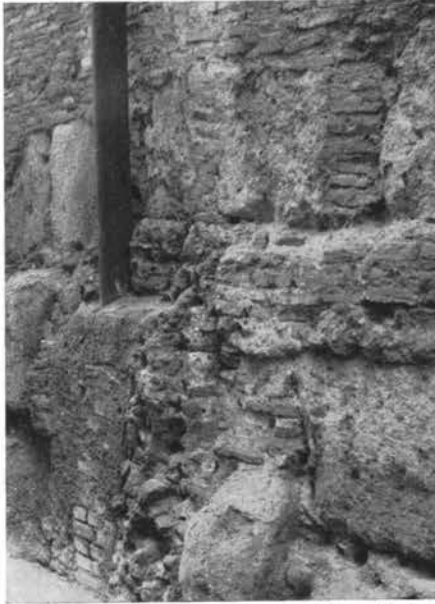
Fig. 96e. S. Martino ai Monti, Ninth century basilica, north aisle, foundation incorporating remains of Roman walls
